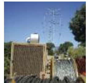
L/Galapagar Junction - S.S. Reyes Junction (Cable laying).
