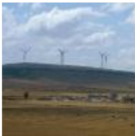
SS. Lora. (Evacuation of energy from the wind farm.)
