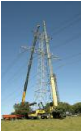
Lifting of support with crane
