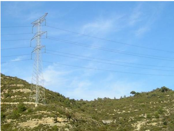
*Most transport power lines ( $\geq 110$  kV) have earth wires on their highest points that intercept lightning; these wires are normally the thinnest and therefore the least visible, and so collision risks increase. Author: Àlex Rollan (CBG-UB).*
