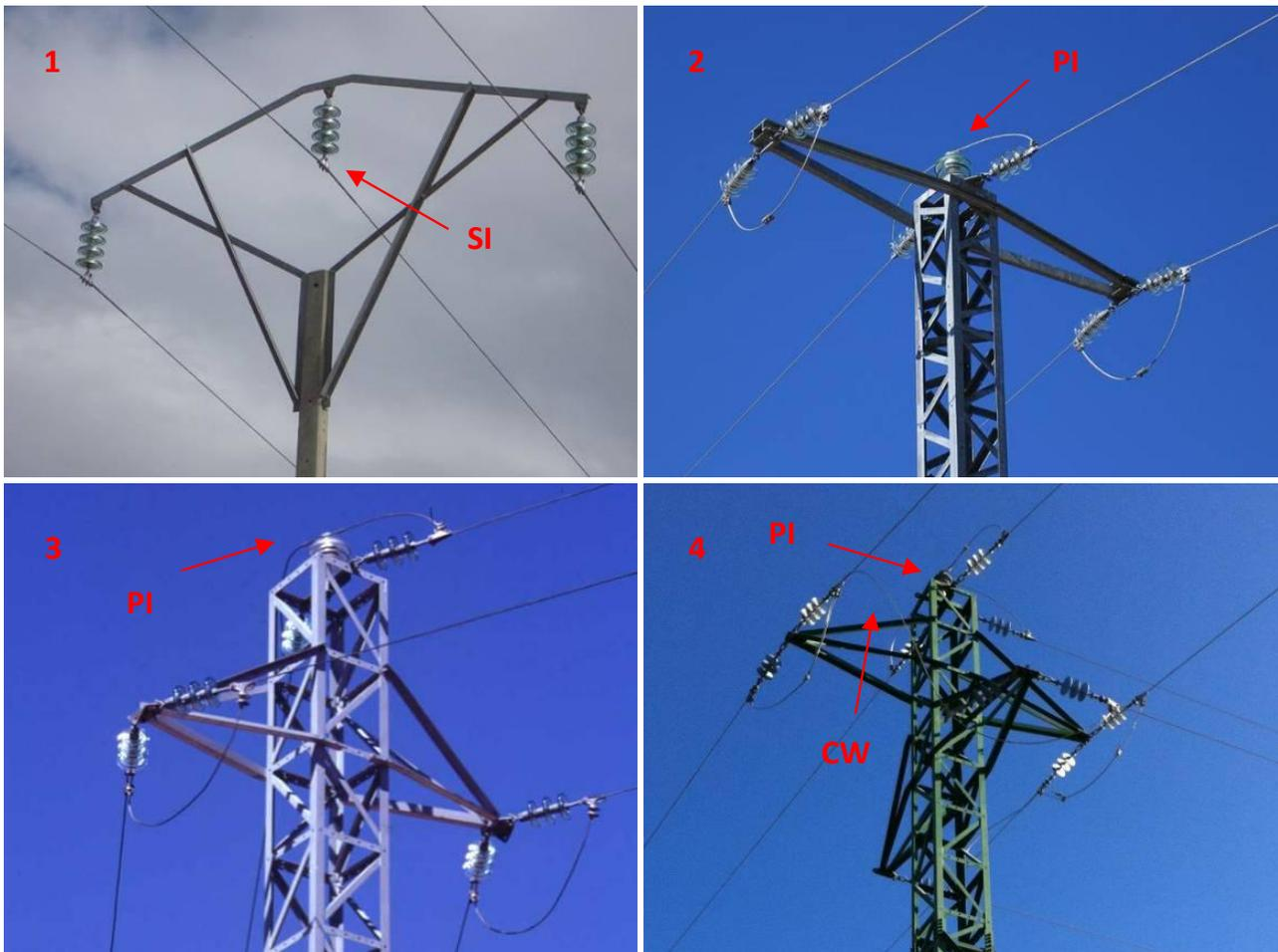
**Figure 23:** Different types of pylons with a high risk of bird electrocution: vault (1), flat (2), cross (3) and perpendicular (4) configurations. Technical elements related to the risk of electrocution are also indicated: suspended insulator (SI), pin-type insulator and exposed jumper (PI), and connector wires (CW). Photos: Albert Tintó (CBG-UB).
